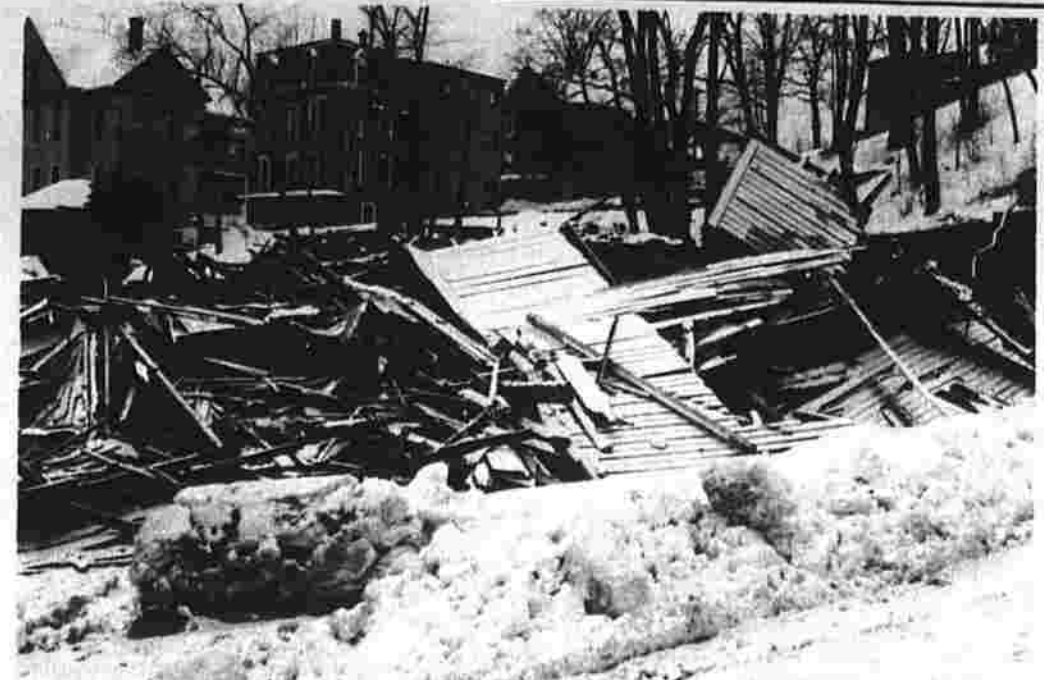
All that remained Friday of a condemned apartment building at 98 W. Main St., Rockville, was a pile of rubble. The building was ordered demolished by the town after it had been extensively damaged by three fires.
